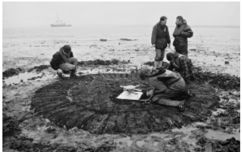
Fig. 4.29: Old cisterns constructed from dried bricks of peat or clay, Wadden Sea north of Pellworm Photo: L. Hermansen
